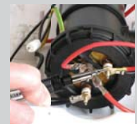
Water Heater Installation
