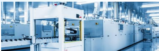
Control Systems PLC, DCS, HMIs, SCADA
