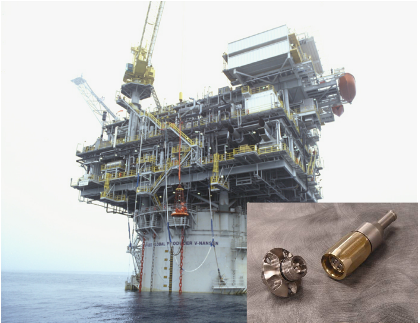
Figure 4. Offshore Production Platform
